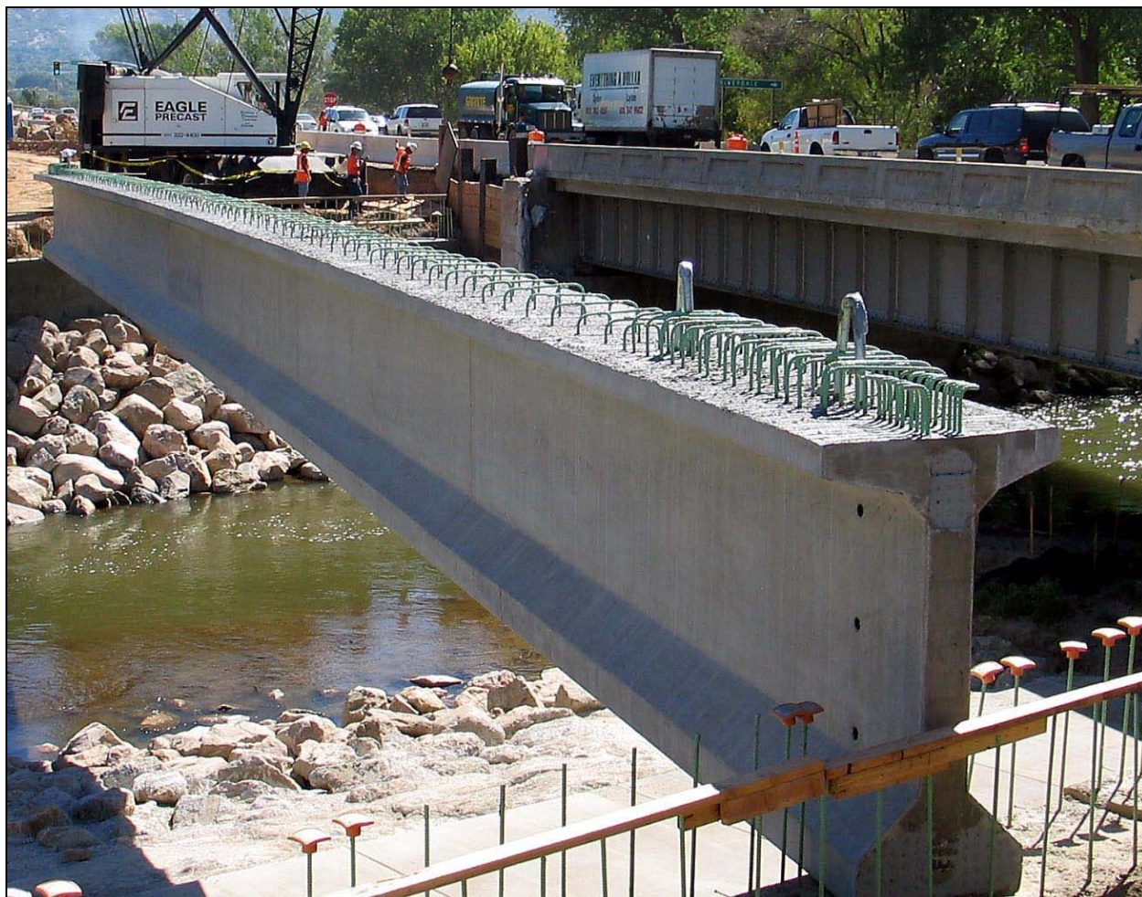
Figure 3. Setting Bridge Girders over the Weber River 26
