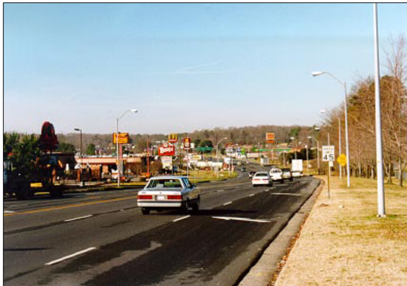
Figure 1. Existing U.S. 64 through Asheboro
